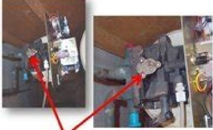
If the softener isn't working try cleaning the filter screen under the metal plate.
